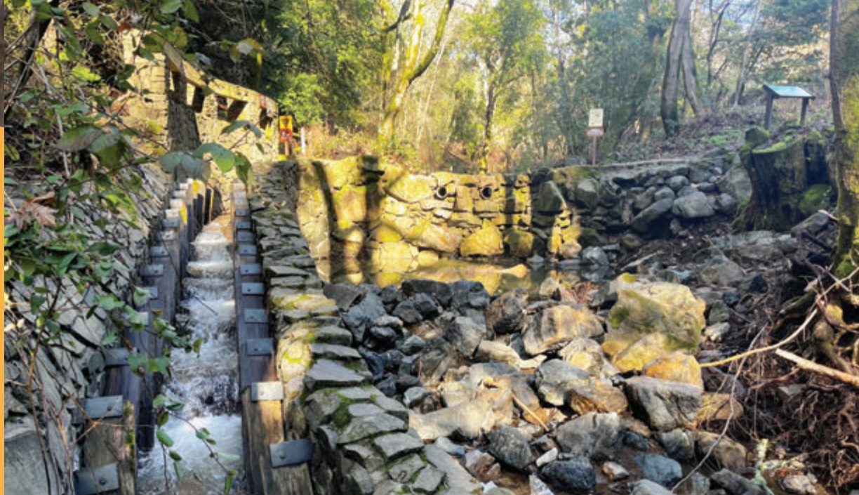
Native trout use a constructed fish ladder to seasonally migrate up Redwood Creek.
